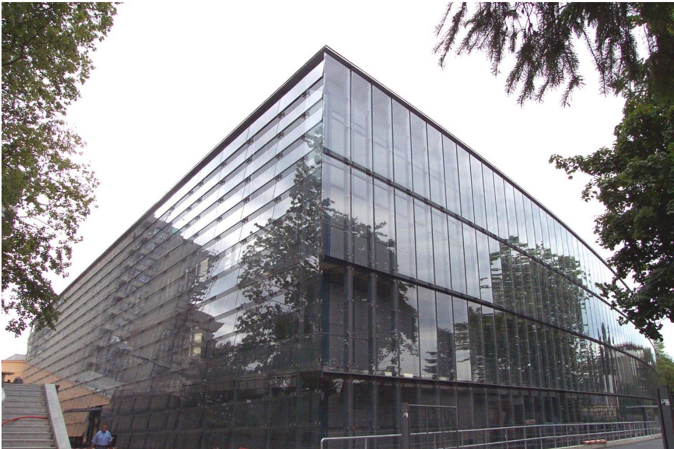
Figure 3, INO (Intensive Care, Emergency, Laboratory and Surgical Center), Inselspital, Bern, Switzerland, Peter Kamm and Kundig, Itten + Brechbühl, 2007-13
