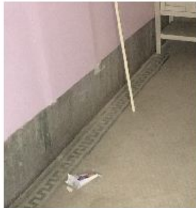
Existing Historic Tile Floor
