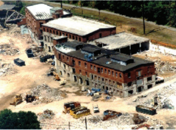
Simpson Paper Mill, Miquon, PA, after partial demolition in 1998.
