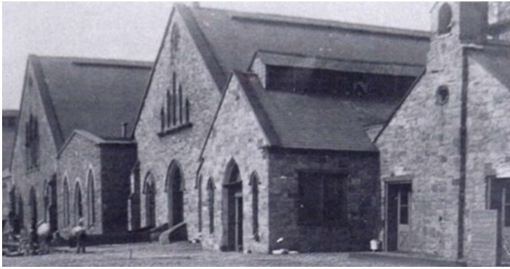
The Purifying Houses of “Church Row” at the Point Breeze Gas Works in 1903. Source: PGW Photograph Collection, City Archives of Philadelphia.
