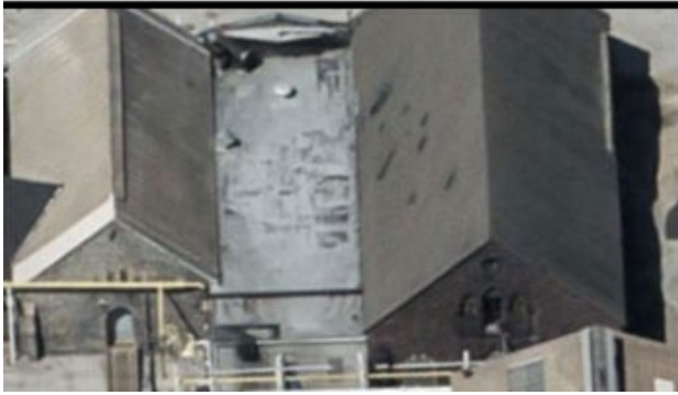
The two Purifying Houses in 2018. Source: Pictometry, Atlas, City of Philadelphia, 2018.
