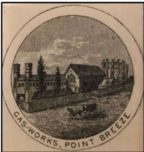
Point Breeze Gas Works in a Strawbridge and Clothier's "Souvenir on Philadelphia," showcasing important architectural landmarks. Source: Historical Society of Pennsylvania.
